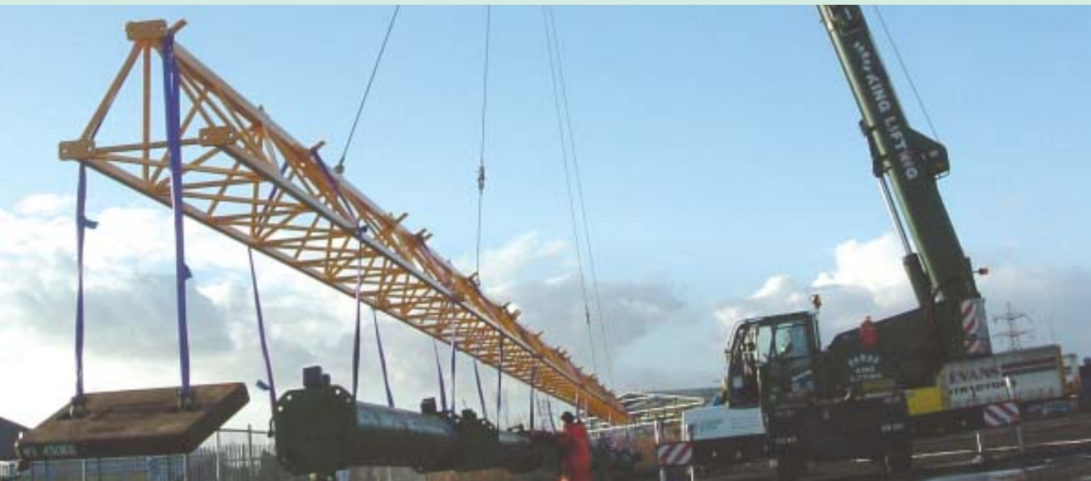
Proof Load Test up to 5 tonnes using the 52.5m Spreader Beam.
